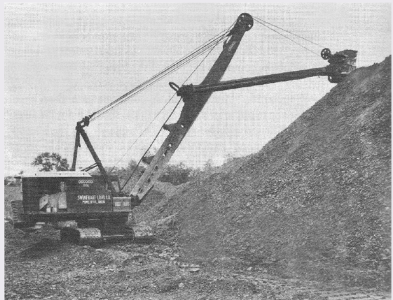
Figure 4. Cable-actuated mechanical shovel manufactured by Osgood General
